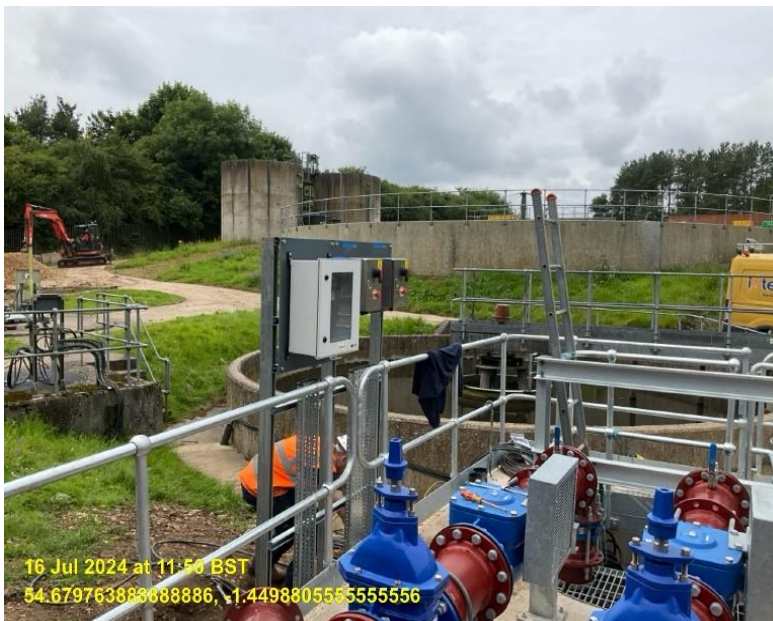
Pumping station being wired up, to allow commissioning.
