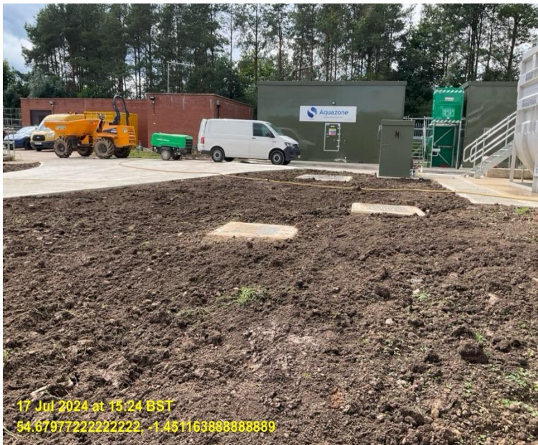
Landscaping works underway, photo of treatment slab
