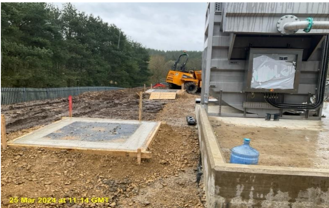
Duct boxes completed with the covers in place:
