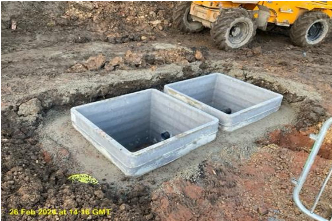
Duct pits installed ready for the covers to be placed:
