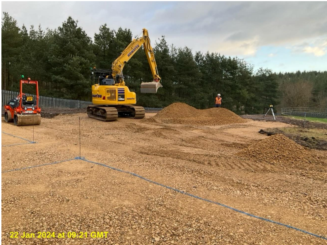
Dosing well underway, fully excavated and now stoning to level.
