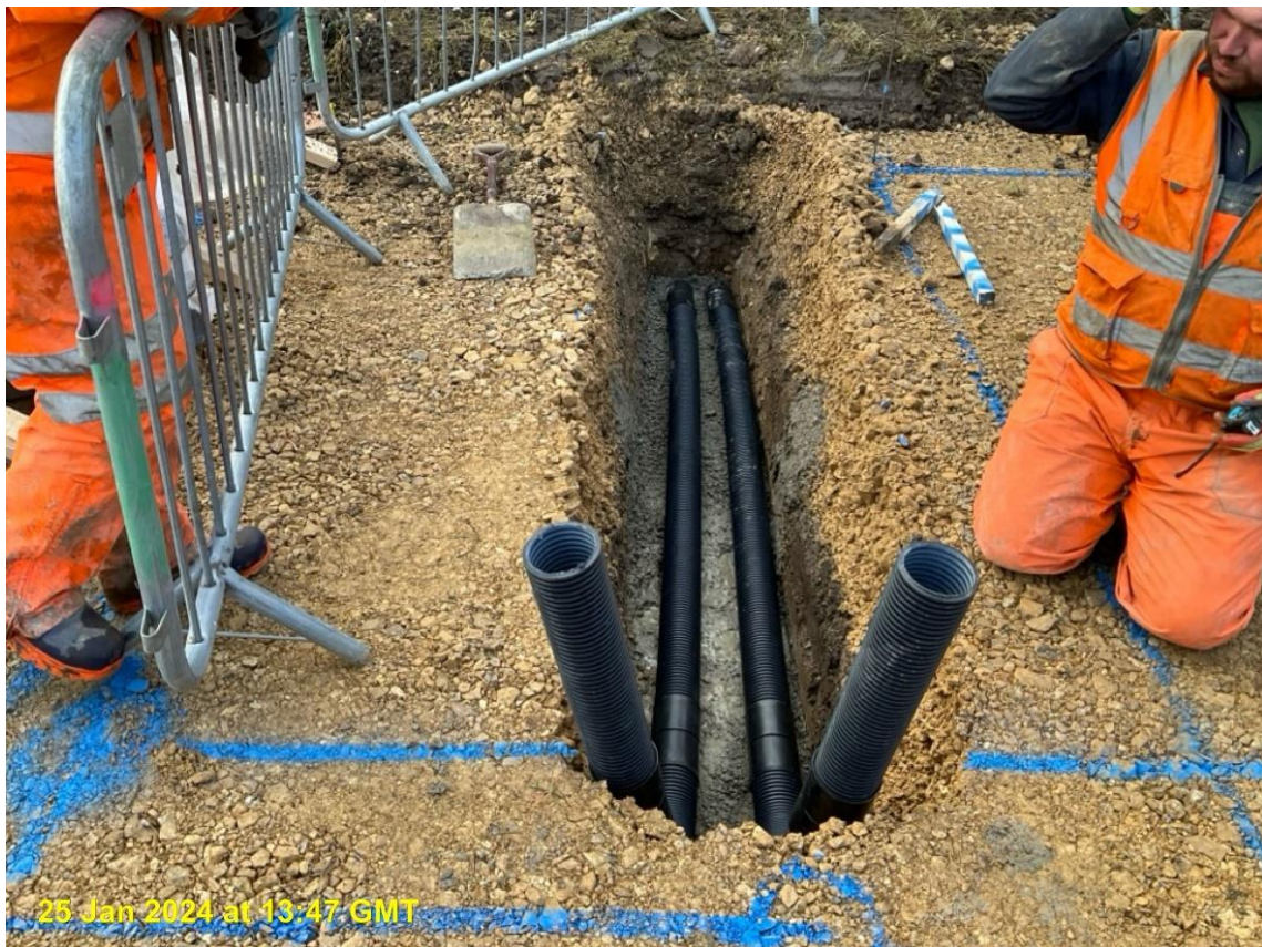
Underground ducting being installed under the proposed dosing kiosks.
