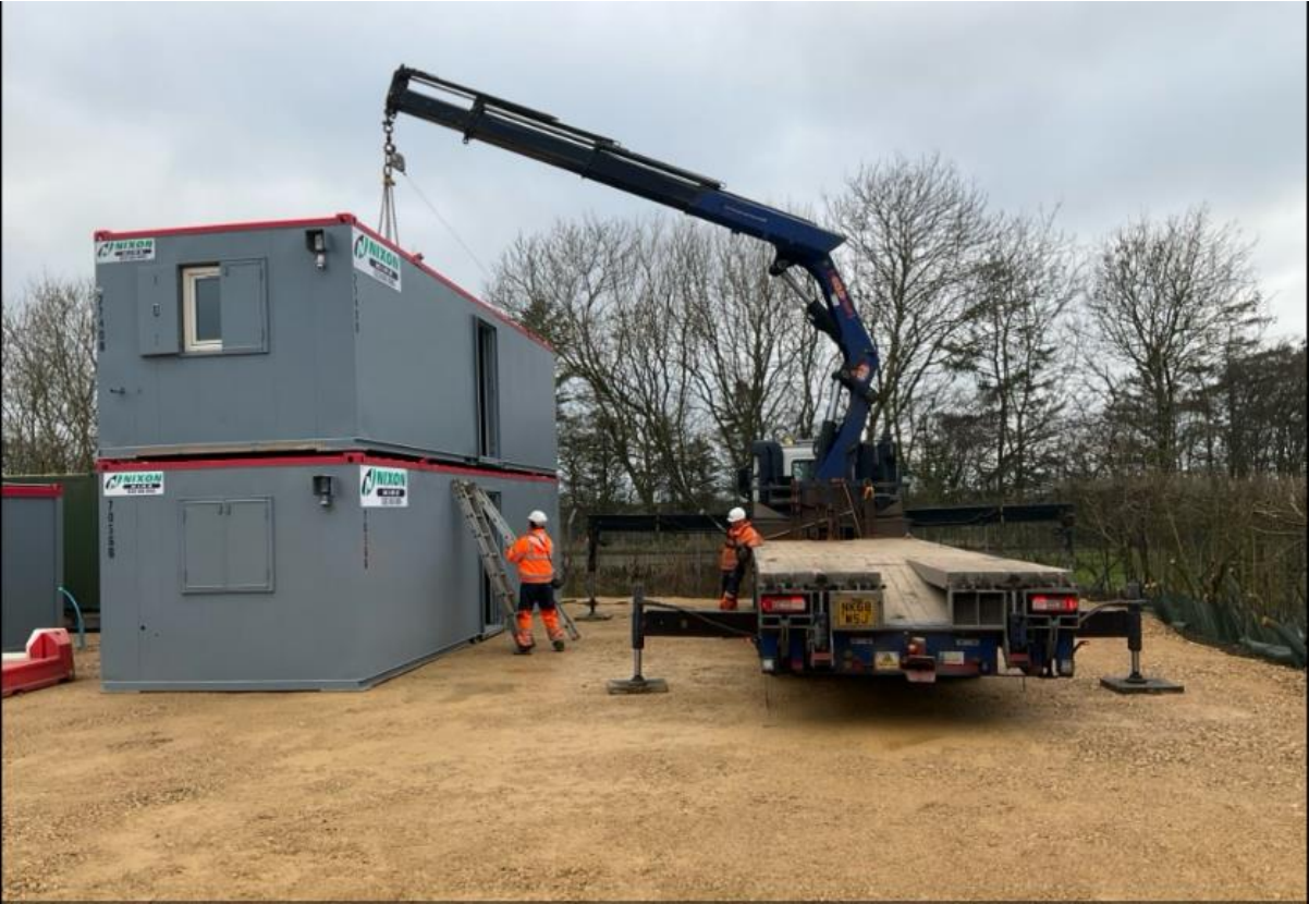
Site welfare units being lifted into position:
