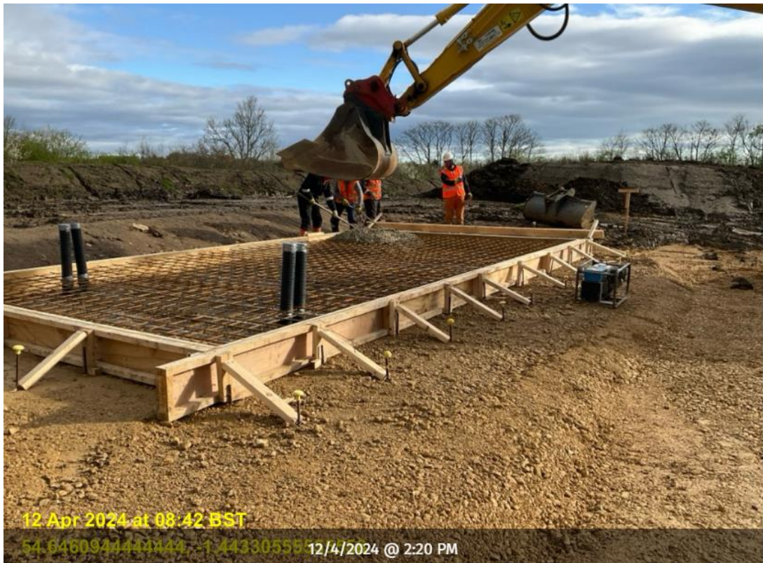
Concrete being laid for dosing kiosks:
