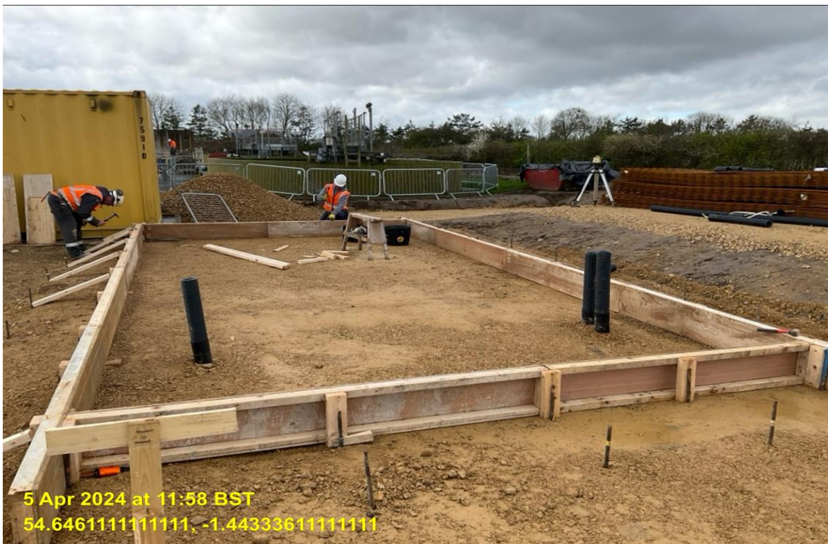
Shutters installed for dosing kiosks:
