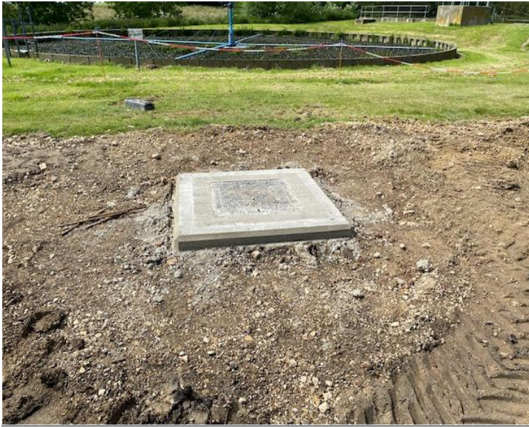
Duct chamber installed
