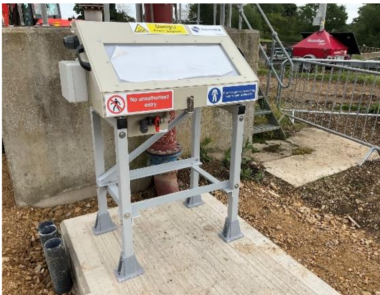
Chemical point of application installed
