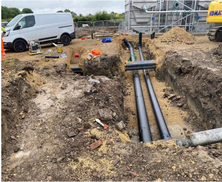
Ducting being installed
