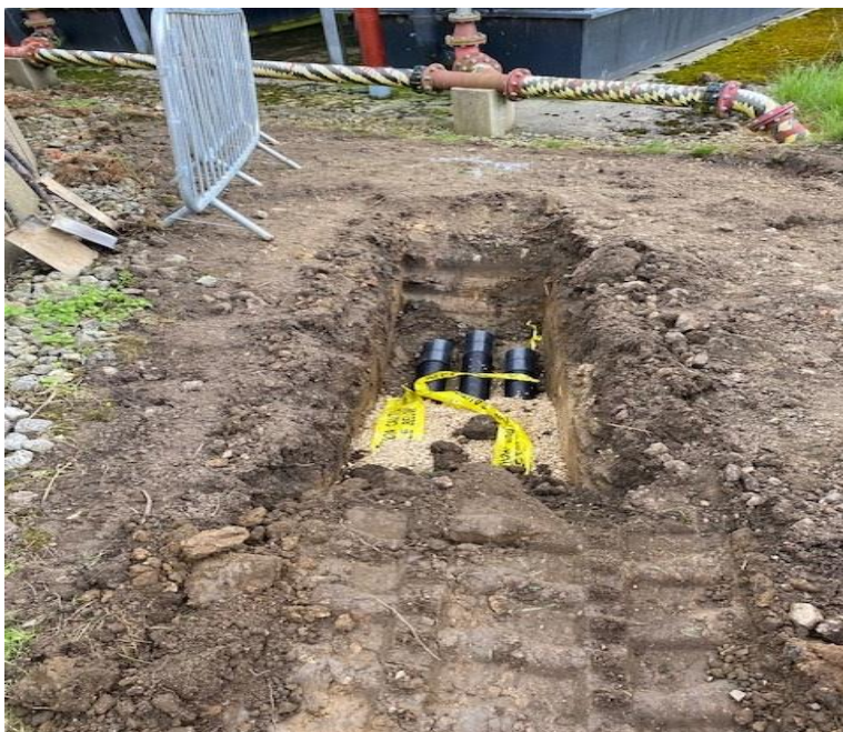
Ducting being installed
