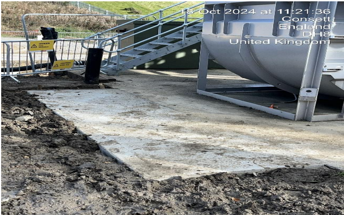
Footway extension to the existing concrete slab at the mecana unit
