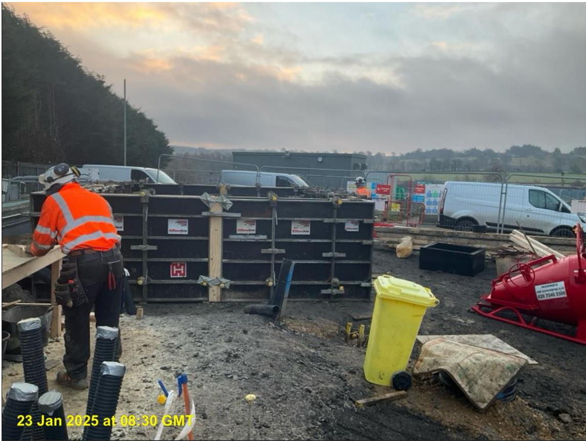
Back wash manhole constructed
