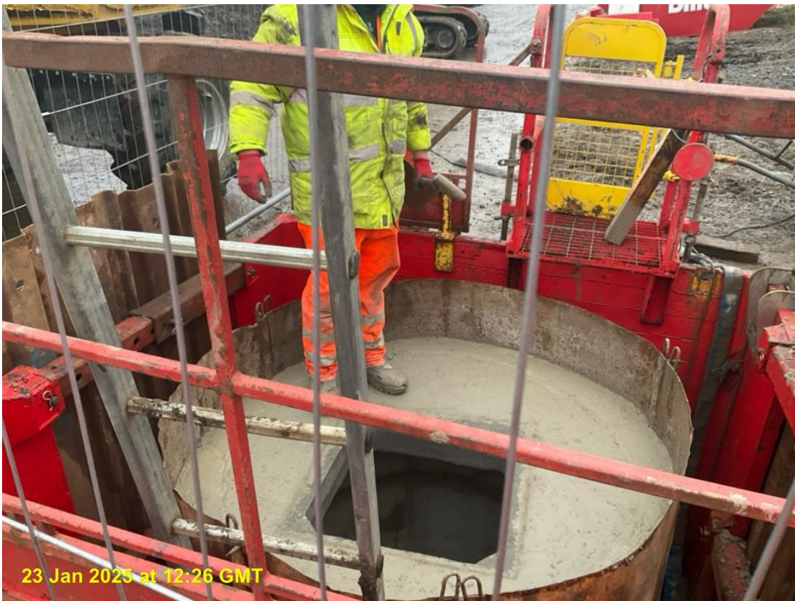
Back wash manhole constructed
