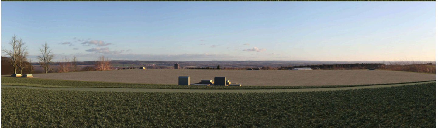
Projected viewpoints from Broom Court (above) and Angel Rise (below), following completion of the project
